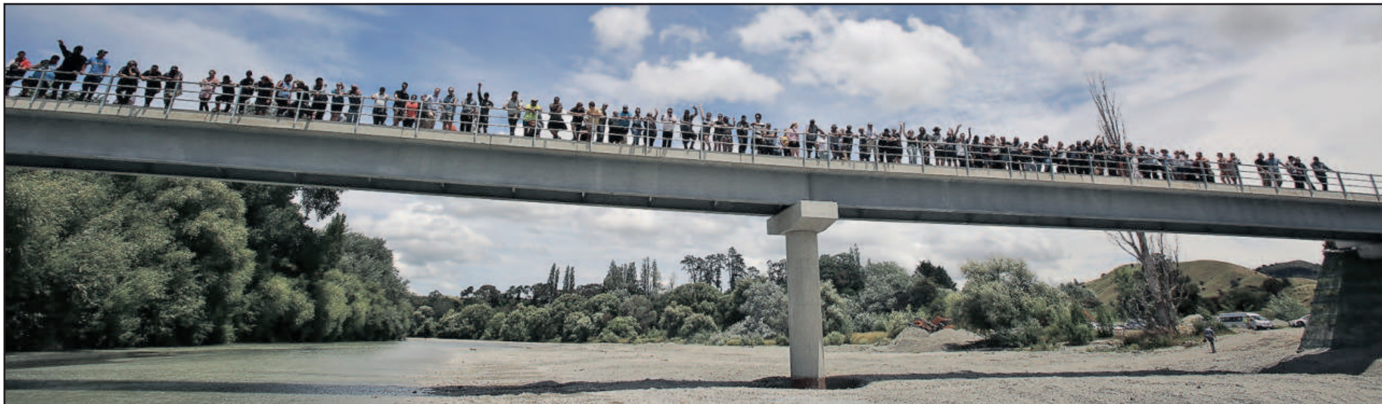
BETTER ACCESS: A new bridge across the Waipaoa River at Whatatutu, built privately by Thompson's Horticulture, improves access to their operation on both sides of the river. The bridge was officially opened by the cutting of a ribbon, and that was done (below) by Marilyn Thompson, pictured with her son Craig (right), who is the company's managing director. They were supported by other family members, staff and their families and others. They all gathered on the bridge (above) after the ceremony. Pictures supplied
